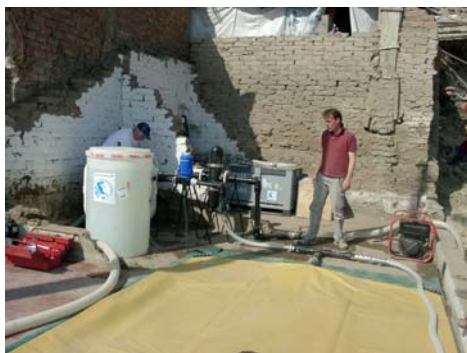
Installation de la mini-station
